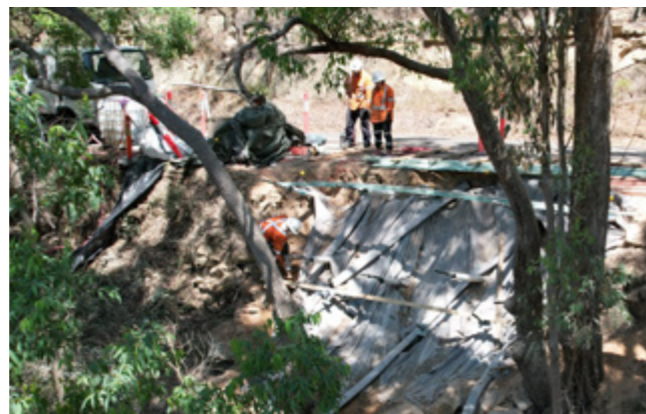
Landslip recovery works at Paynes Crossing Road
