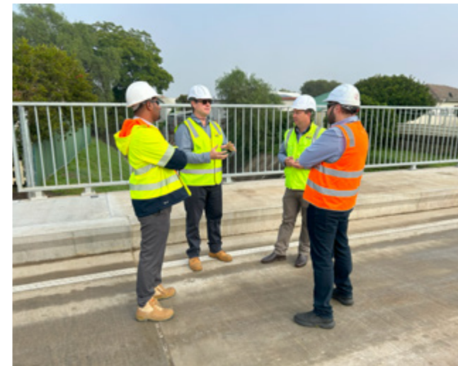
A new bridge for Kline Street, Weston
