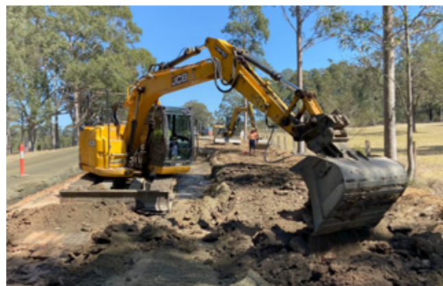
Upgrades to Sandy Creek Road, Quorrobolong
