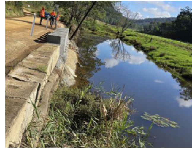
Embankment stabilisation for Murrays Run Road, Murrays Run
