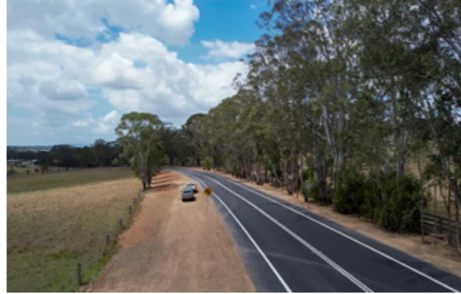
Improved road condition for Wollombi Road, Millfield
