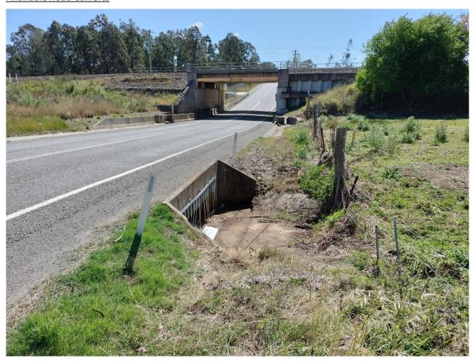
Dimensions: 1 x 2.4m wide x 0.6m high box culvert
