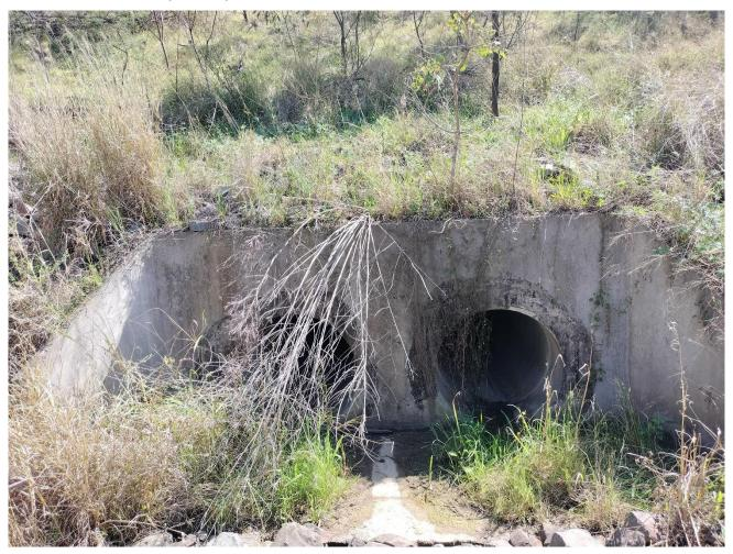
Dimensions: 2 x 0.9m diameter pipes
