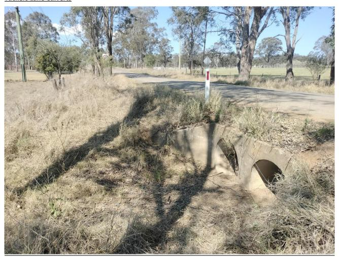
Dimensions: 2 x 0.9m diameter pipes
