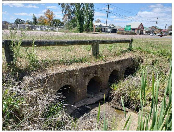
Dimensions: 4 x 0.6m diameter pipes
