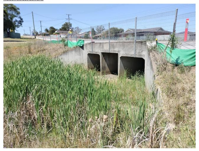
Dimensions: 2 x 2.1m wide x 1.8m high box culverts and 1 x 2.1m wide x 1.9m high link slab
