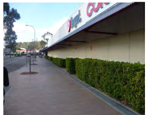
Figure No 20: Blank walls to streets.
