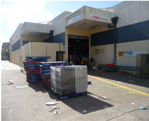
Figure No 23: Exposed 'back of house'
