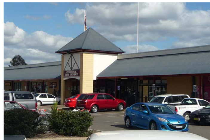
Figure 93: Site 3 - Coles Supermarket Site
