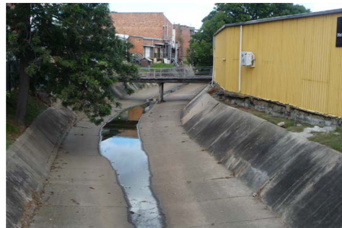
Figure 97: Site B - Stormwater Canal (north)
