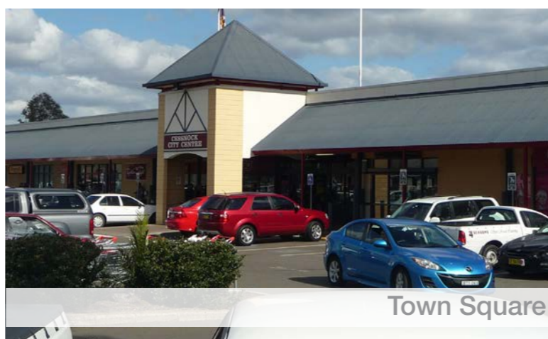
Figure 33: Existing Cessnock City Centre
