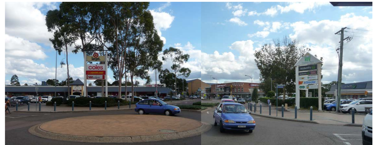
Figure 124: Roundabout impacts upon pedestrian access along Cooper Street.
