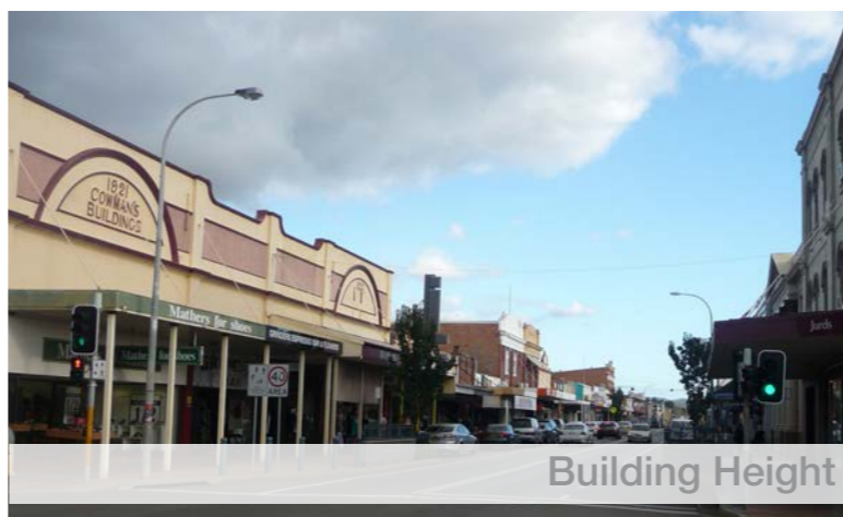
Figure 34: Existing Intersection of Vincent Street and Cooper Street
