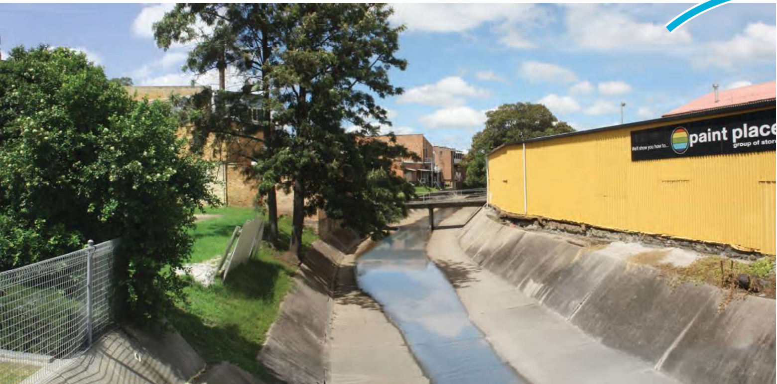
Figure 29. Drainage channel at the northern gateway - existing situation
