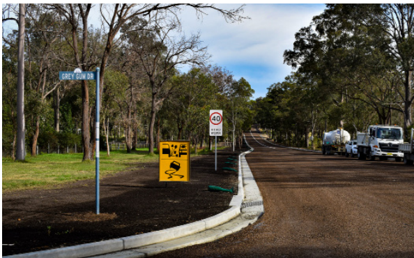
Photo : Gingers Lane Roadworks
