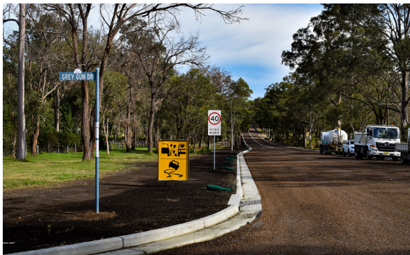
Photo : Gingers Lane Roadworks
