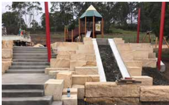
Photo: Bridges Hill Playground, Cessnock (March 2019 progress)
