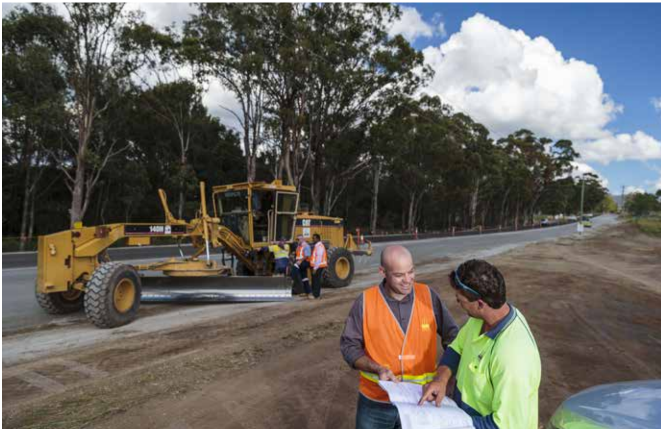
Cessnock Council road construction
