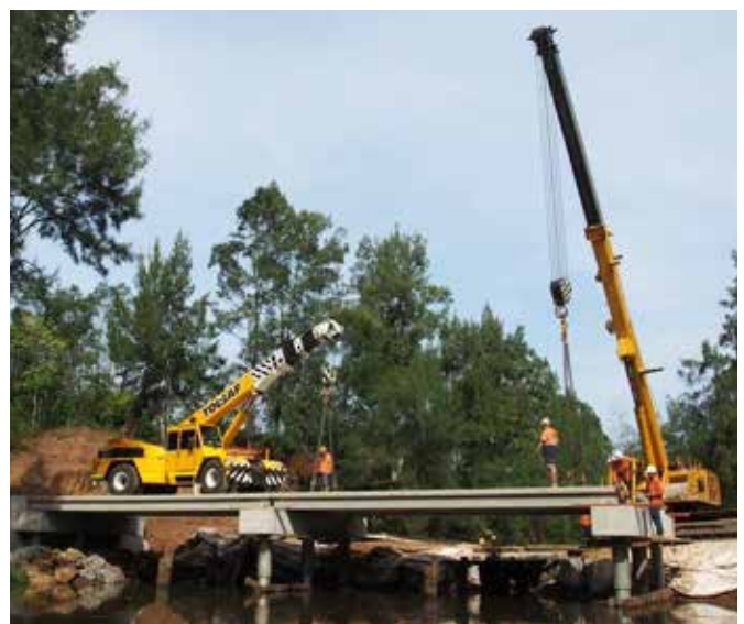
Williams Bridge Construction
