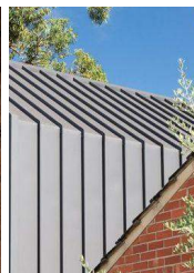
GREY METAL DECK ROOF
