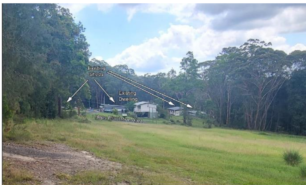
Figure 3 – View of existing structures located on the site
