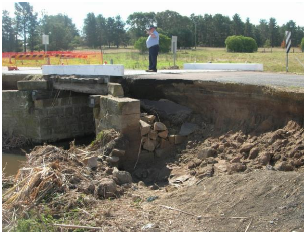
Photo 3: Branxton Street Bridge 2015
