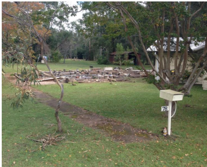
Photo 8: 78 Sale Street, Greta – House knocked off foundations, 2015
