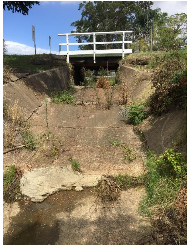
Photo 25: Hunter Street - steep gradient drop directly downstream of the hydraulic structure
