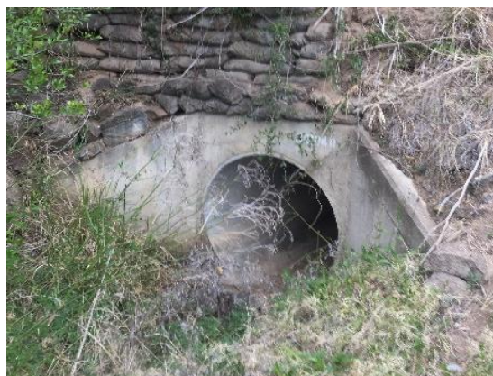
Photo 28: Road Culverts underneath New England Hwy, Greta
