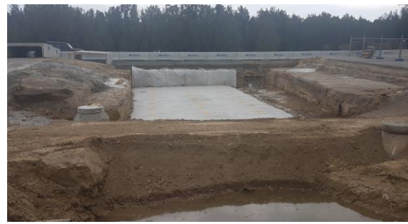
Photo 30: Construction at the New England Highway
