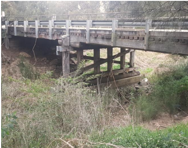
Photo 26: Nelson Street Bridge
