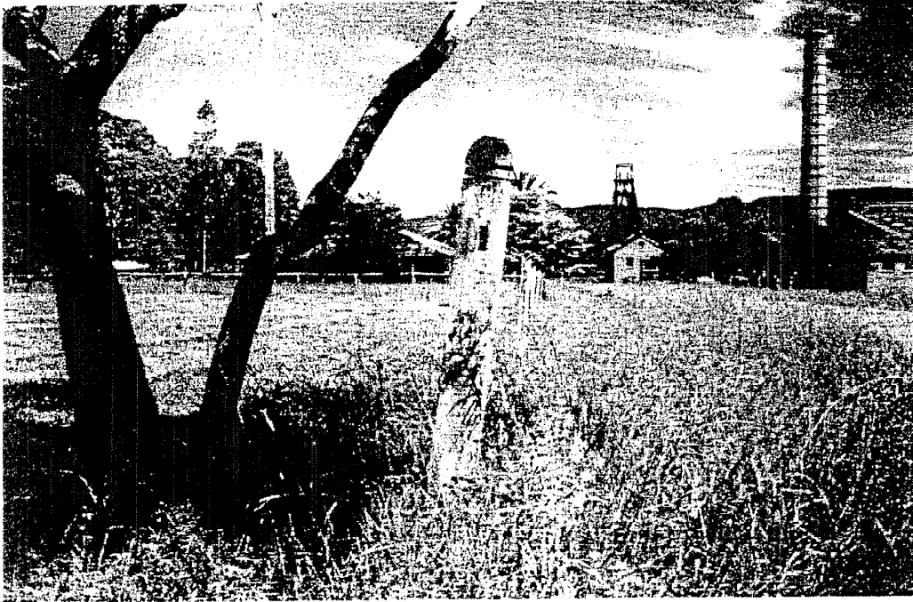
FIGURE 4.12: FENCE POST TO MECHANICAL ENGINEER'S COTTAGE
