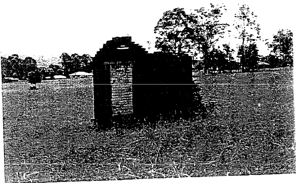
Photograph Four View of the explosives store from the south-west. The site was selected by the Millfield police officer in 1922 (Hunter 1999).
