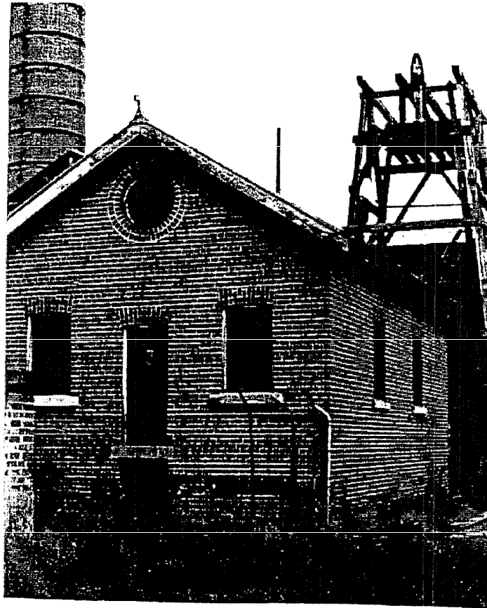
Photograph Eleven The winder house, for the upcast shaft, from the north.
