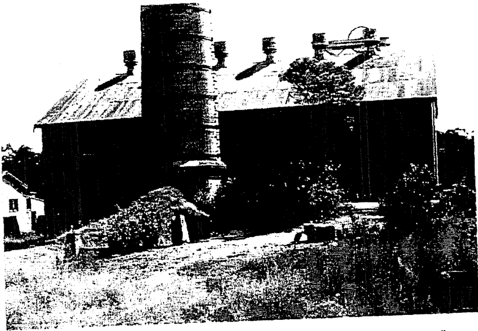
Photograph Fifteen View of the power house, stack and covered boiler house floor from the east.
