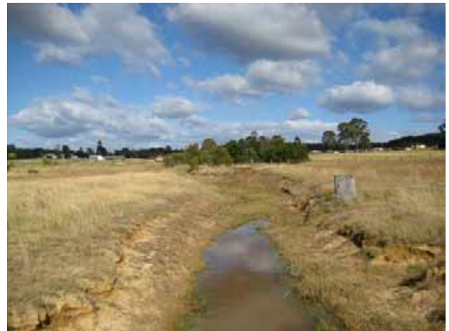
Bellbird Creek Tributary 1– showing no remnant species, and constructed, degraded channel
