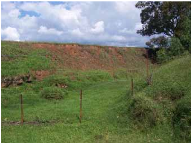
Limestone Creek channel showing significant height of banks at meander bends
