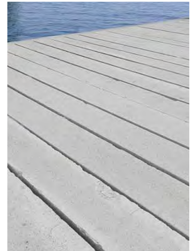
Concrete suspended plank pavement
