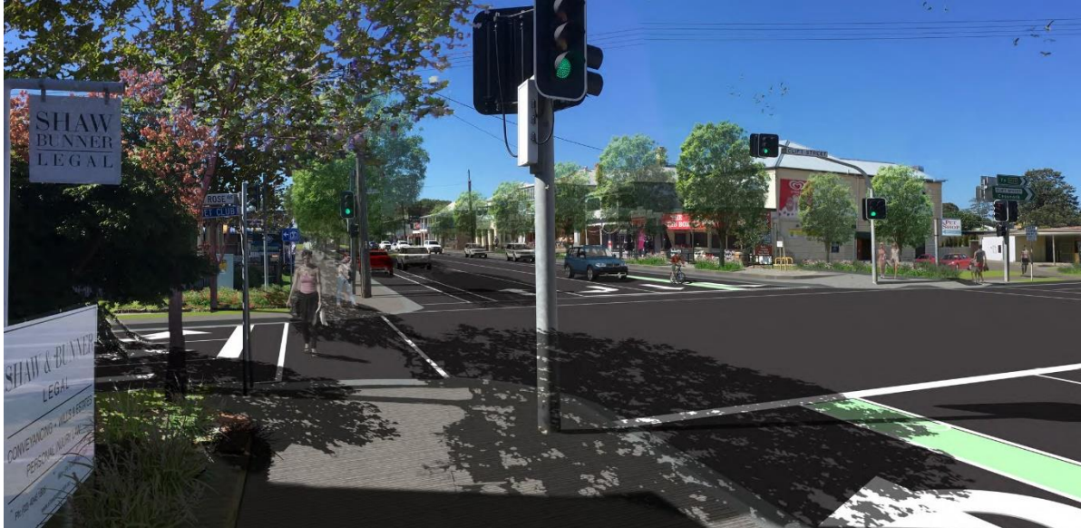
Figure 3: The intersection of Maitland and Clift Streets and John Rose Avenue, Branxton.
