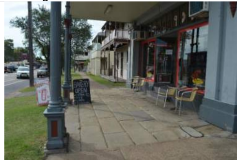
Photo 6: Main street with verandas and other heritage paving features
