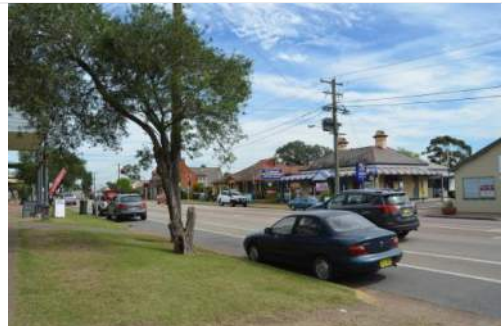
Photo 12: Existing northern frontage
