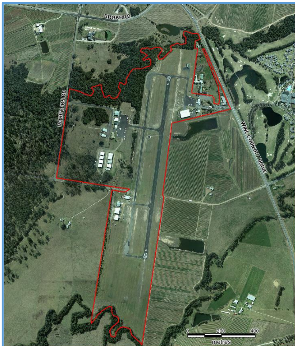
Figure 1: Aerial of Cessnock Airport - 2018
