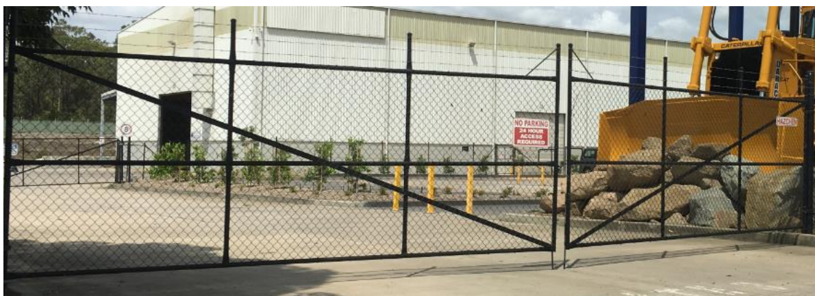
Figure 6 – Black chain wire fencing along secondary, side and rear boundaries.
